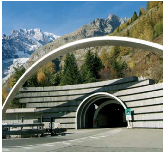
Tunnel Monte Bianco - Mont Blanc Tunnel
